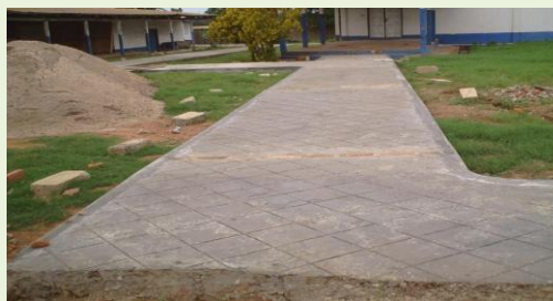
A new paved walkway
